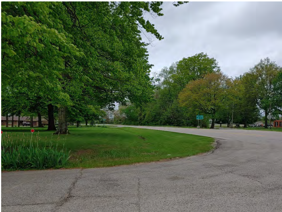
25. Looking west along West Fuson Road from the intersection of South Edgewood Drive and West Fuson Road.
