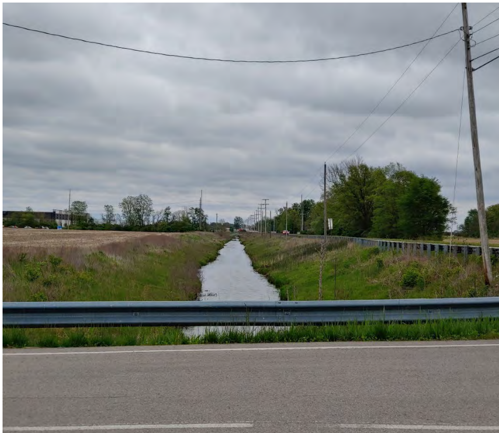
27. Looking east along the drainage channel north of West Fuson Road and east of South Delaware Drive.
