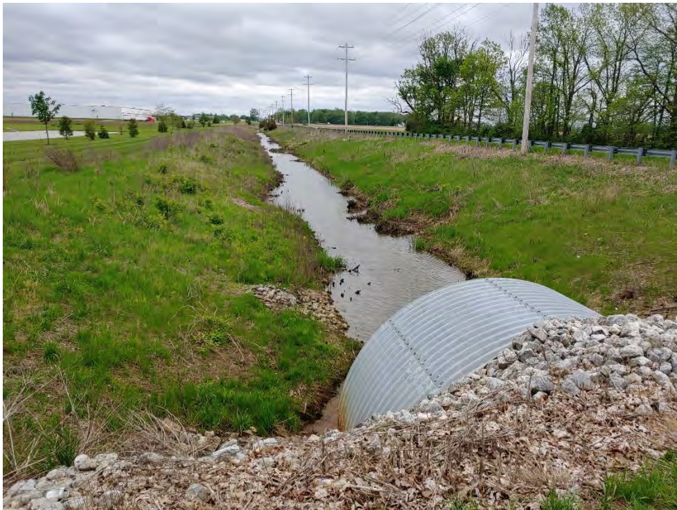
29. Looking east at a culvert crossing of the drainage ditch north of West Fuson Road. Photograph taken at a location east of South Delaware Drive and West of South Cowan Road.
