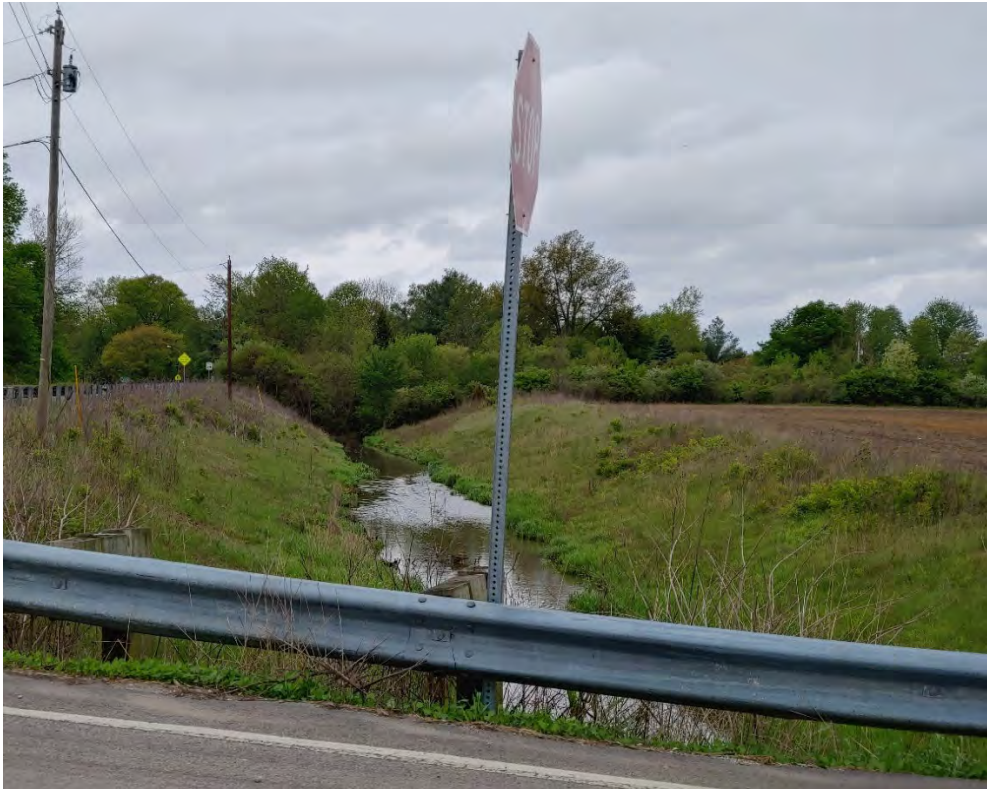
28. Looking west along the drainage channel north of West Fuson Road and west of South Delaware Drive.
