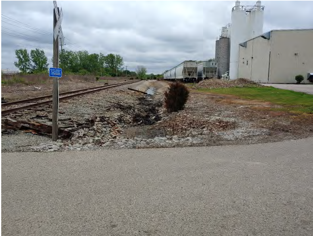
10. Looking east along the north portion of MUNDELL ID M45 from South Niles Road.
