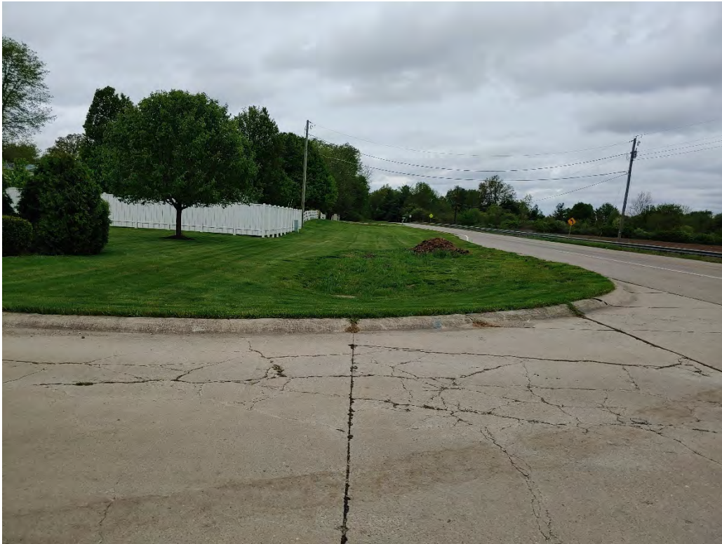
22. Looking west along West Fuson Road taken at the intersection of South Delaware Drive and West Fuson Road.
